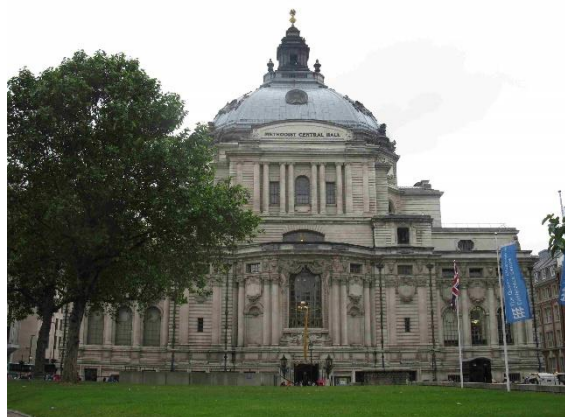
Methodist Central Hall
